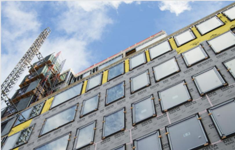
24 2<sup>nd</sup> Avenue needed an advanced weather-resistive barrier that contributes to a high-performing, energy-efficient building
