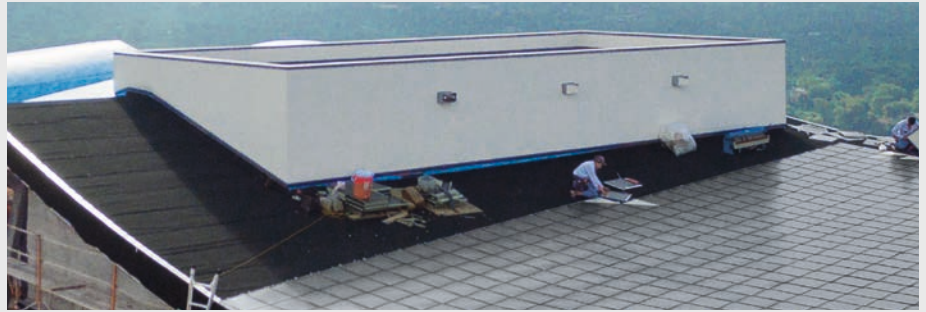
Installing the 2500 panel roof.
