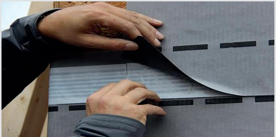
"This specification establishes the test methods and minimum performance requirements for self adhering flashing products that are used around the perimeter of exterior fenestration products. It also provides a method to determine the minimum width of the flashing products and to evaluate the influence of the environmental factors on the installation of self adhering flashing products applied under typical field conditions" (AAMA 711-07)
