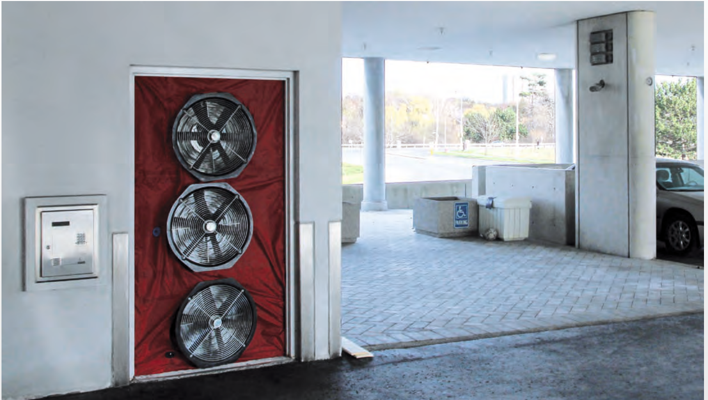
Typical blower door test at multi-story building
