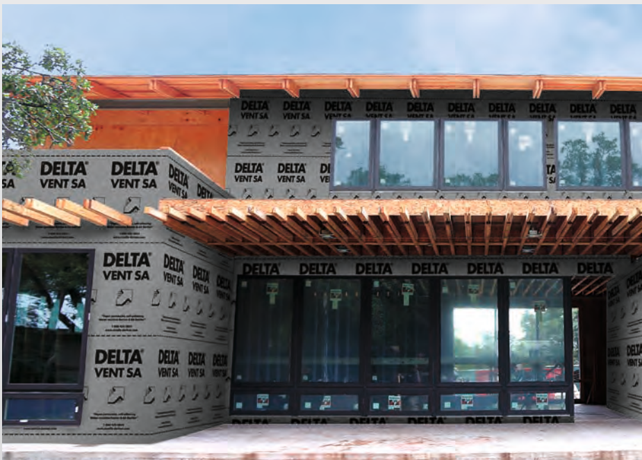
Air barrier application in residential construction
